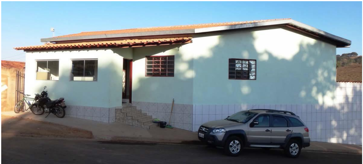
Figure 11.5-1 VERDE Office and Sample Storage Yard/Preparation Area (Matutina) (August 2012)
