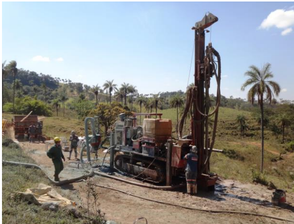
Figure 10.4-3 RC Drilling #2 - CV Target 7 (August 2012)
